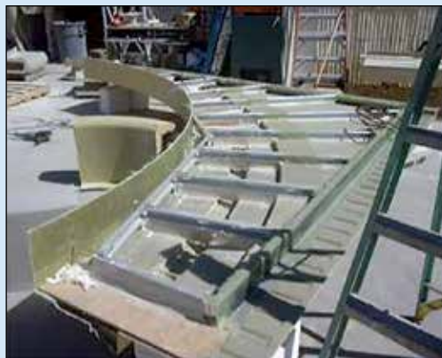
FIGURE 5.6-1: Stiffeners attached to backside of an E-glass FRP panel
